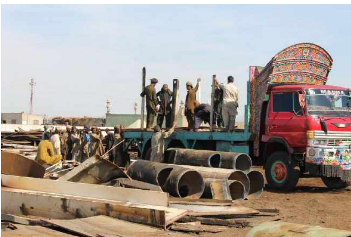
Below: Workers load steel bars onto the trucks
