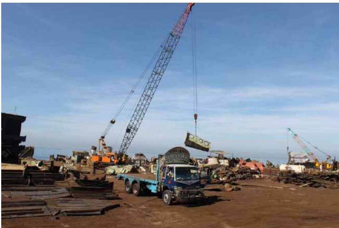
Above: Cranes load the heavy steel parts onto the trucks for delivery to the recycling plants
